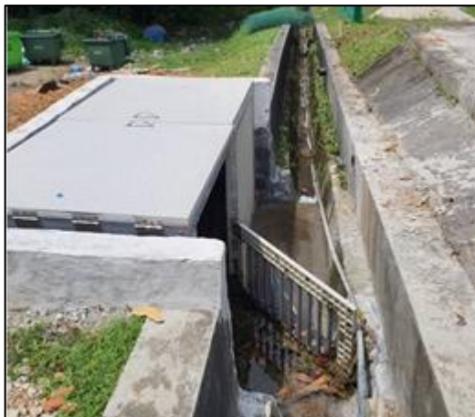
Fig. 1. Waste trap in the drainage system
